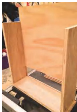
STEP 17. Next, insert a 6mm panel for the bottom
